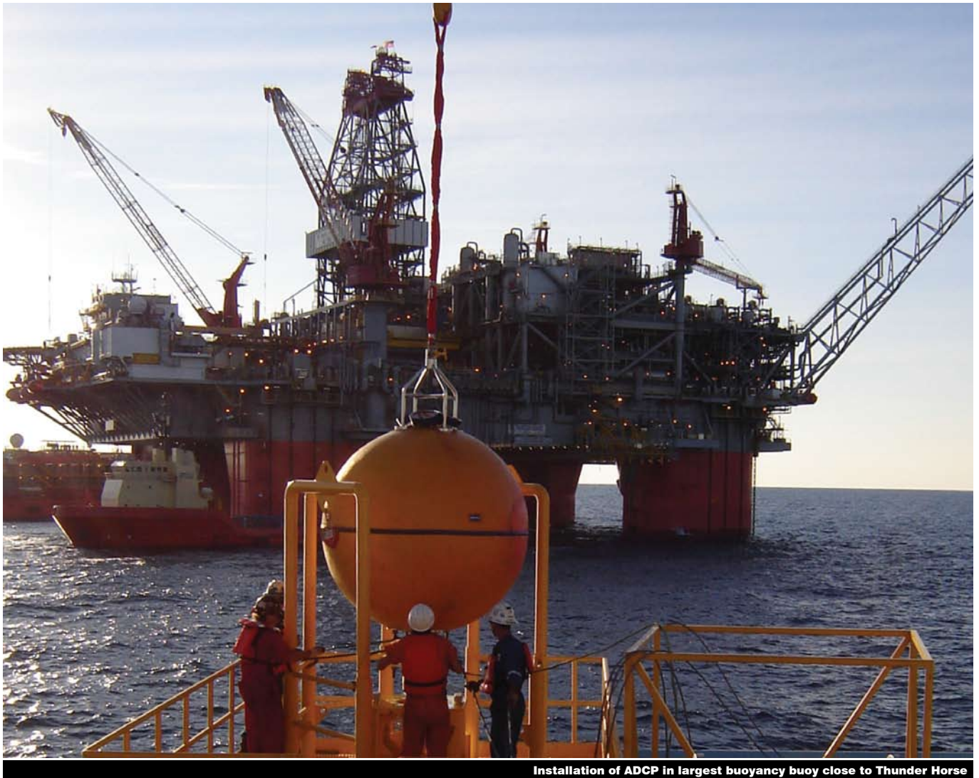
Installation of ADCP in largest buoyancy buoy close to Thunder Horse
